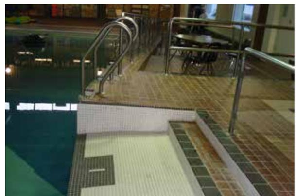
Photo 4: Lose hand railing in shallow end of the pool
