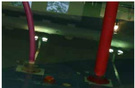
Photo 18: Paint peeling on water features
