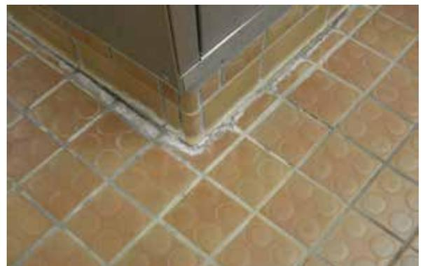
Photo 6: Cracked tiles in the female change room
