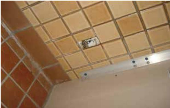
Photo 7: Cracked tiles in the female change room
