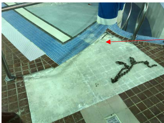
Photo 9: Tile Removal Area H
