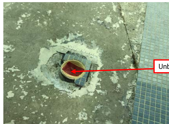
Photo 7: Control joint at Tile Removal Area G Photo 8: Unbonded grout at Tile Removal Area G
