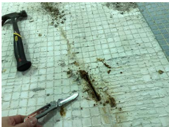
Photo 7: Control joint at Tile Removal Area G Photo 8: Unbonded grout at Tile Removal Area G
