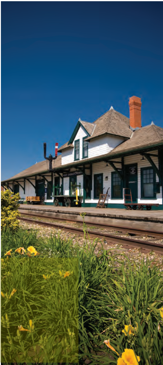
CN Station, Fort Saskatchewan
