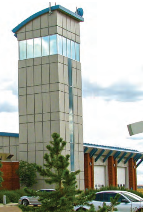
Station #4 Heartland Hall, Strathcona County
