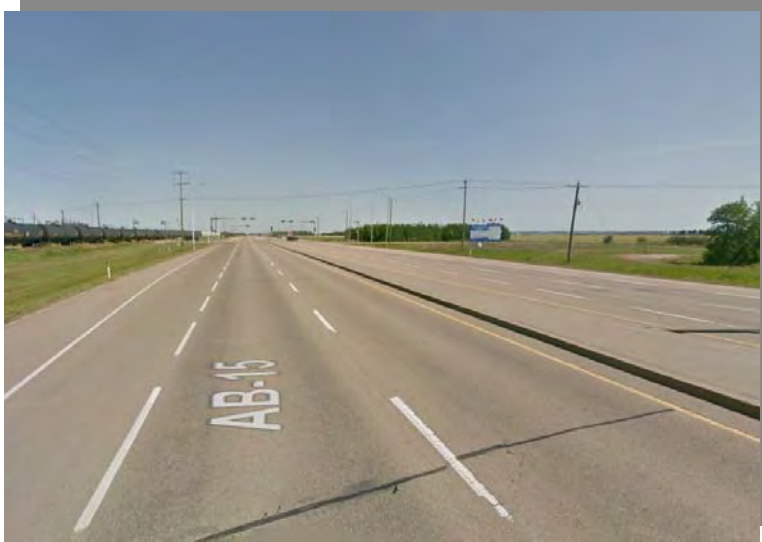
Photo 1: Highway 15 west of 125 Street – Looking East
