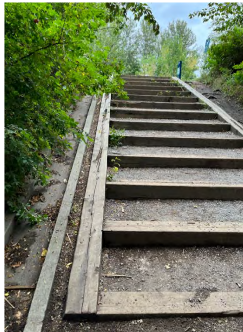
Image of earth-embedded staircase
