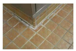
Photo 6: Cracked tiles in the female change room
