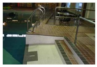
Photo 4: Lose hand railing in shallow end of the pool
