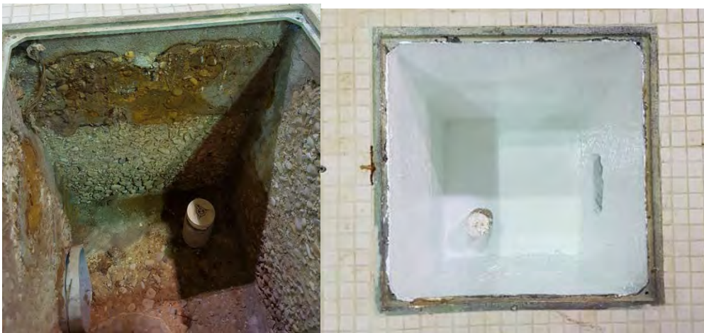
Harbour Pool main pool floor drains concrete repairs and epoxy coating before and after.
