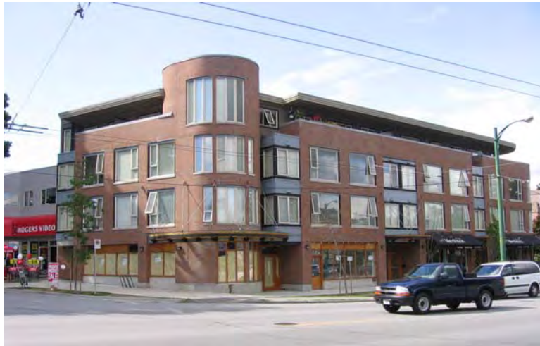
This corner lot fronts both the street and the avenue. The roof line of the building is architecturally articulated and the entrance to the ground floor is highlighted through the use of a canopy, emphasizing a distinguishable retail establishment.
