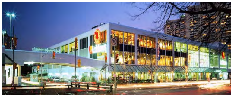
The large tenancy in this building is located above smaller tenancy frontages that are highly transparent. Entrances to smaller tenancies are provided at intervals of 6.0 - 10.0 m.
