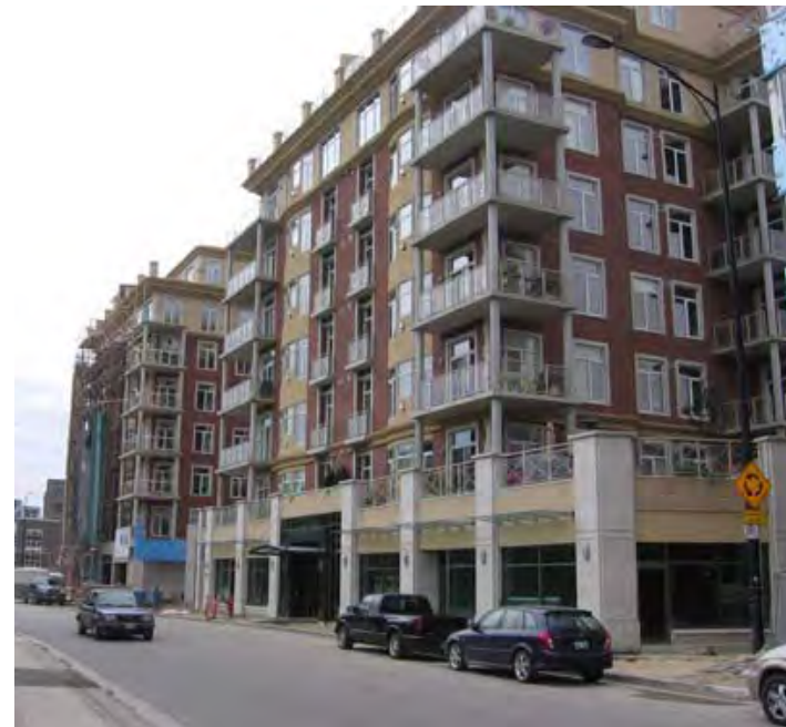
The balconies project a maximum of 1.0 m from the building face. An outdoor terrace above the ground floor provides additional amenity space for occupants.
