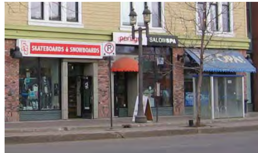
The entrances to this building are facing the adjacent street, universally-accessible, and are clearly indicated through the use of canopies and other signage.
