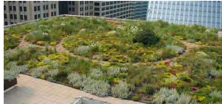
A rooftop garden increases rainwater permeability and filtration, while reducing energy consumption and the urban heat island effect.
