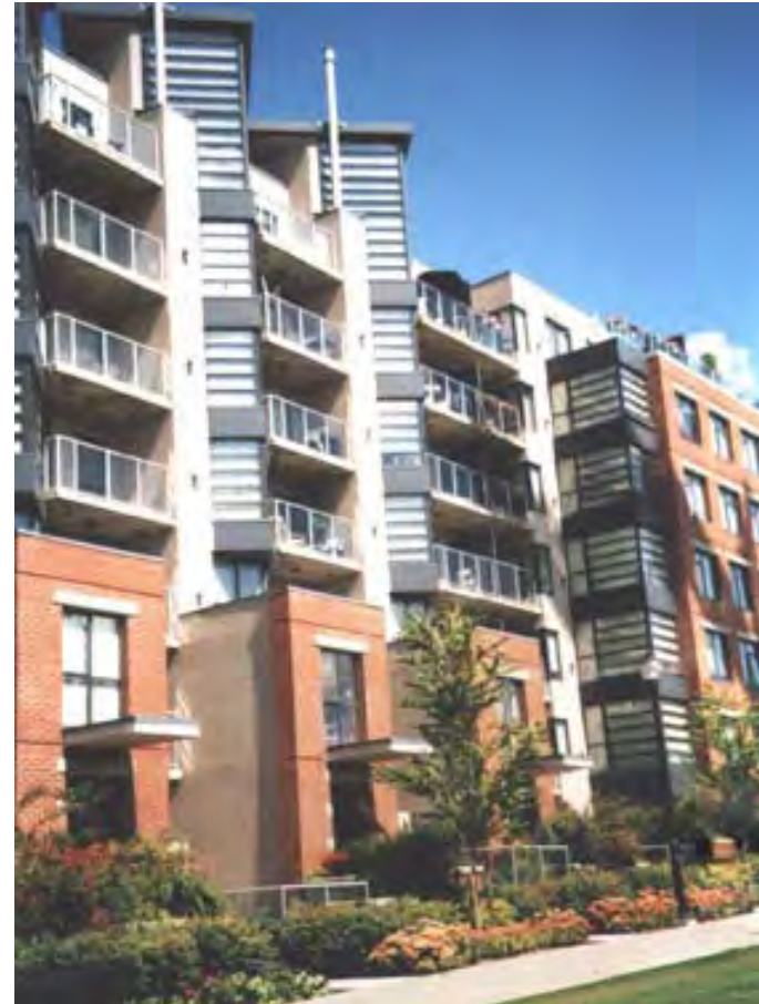
The balconies of this building are an integral part of the structure and do not seem “tacked” on. Outdoor terraces on the roof top provide additional amenity space for residents.
