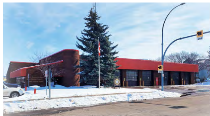
CITY OF FORT SASKATCHEWAN FIRE STATION #1
