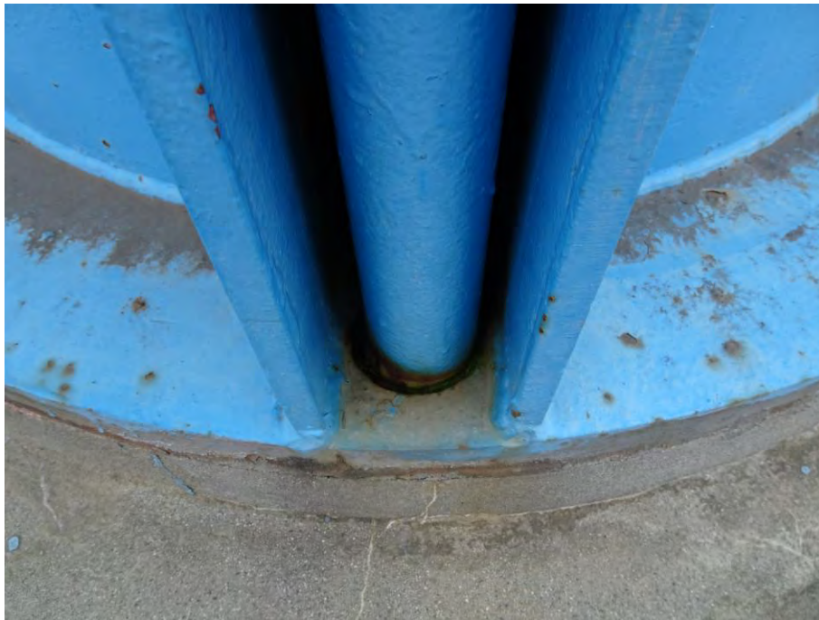
Photo S-7: Anchor bolts at column baseplate (Pier #5)
