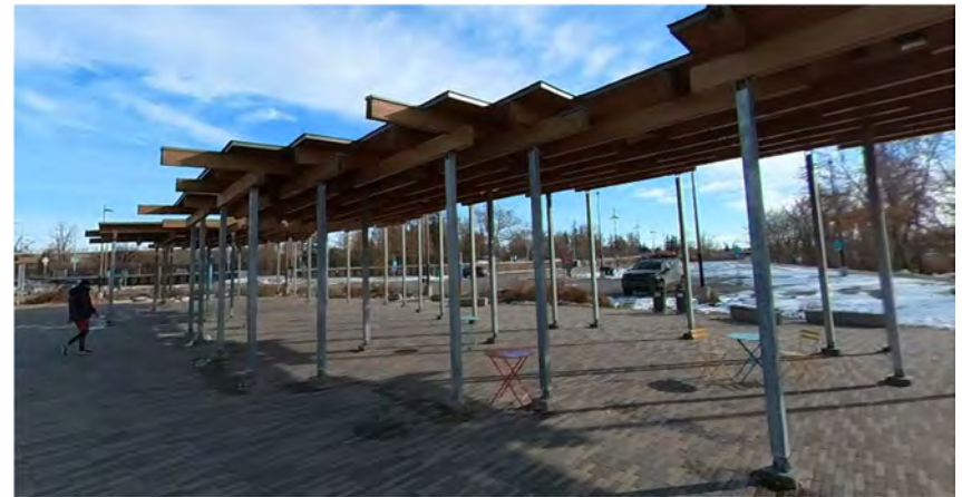
Multi-Purpose Public Covered Plaza, Calgary, AB (Source: Google Maps)
