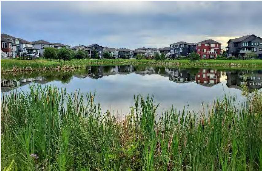
Naturalized Stormwater Management Facility (Source: Strata Development Corp)
