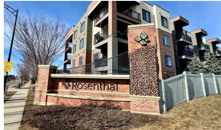
Entry Feature Example (Source: Strata Development Corp.)
