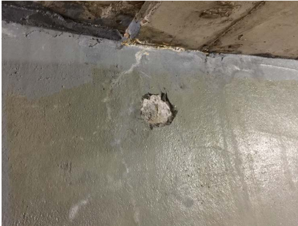
Photo 11: Main pool deep end wall from below grade corridor – cementitious material applied onto wall
