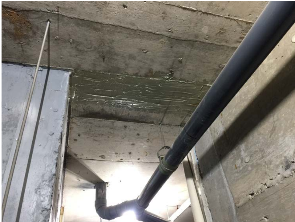
Photo 22: Epoxy filler at crack location on underside of pool deck
