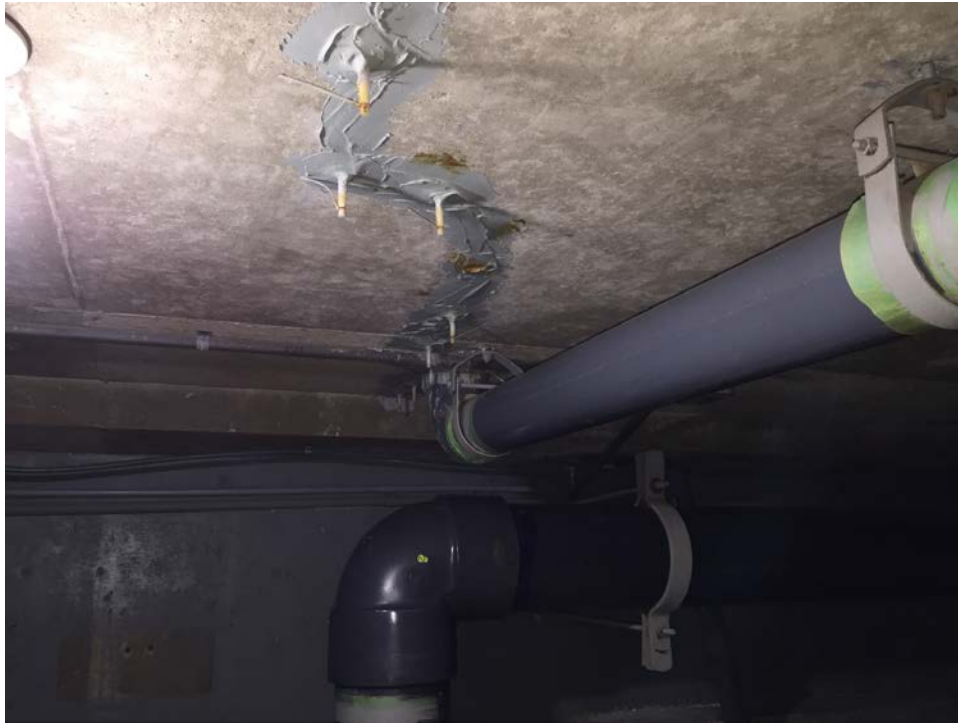
Photo 21: Crack injection at pool deck drain
