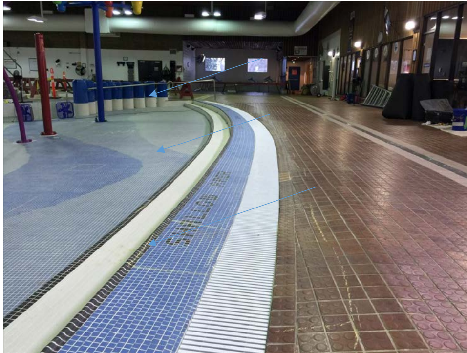
Photo 15: Pool deck and trench drain
