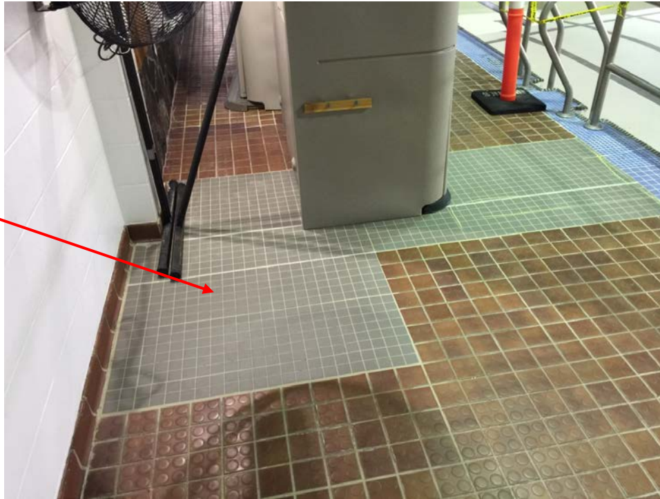
Photo 19: Tile replacement on pool deck
