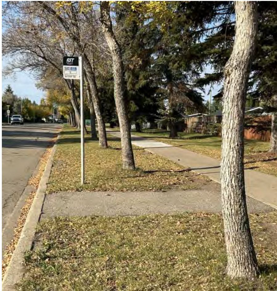
Figure 1 - Current bus stop with asphalt pad
