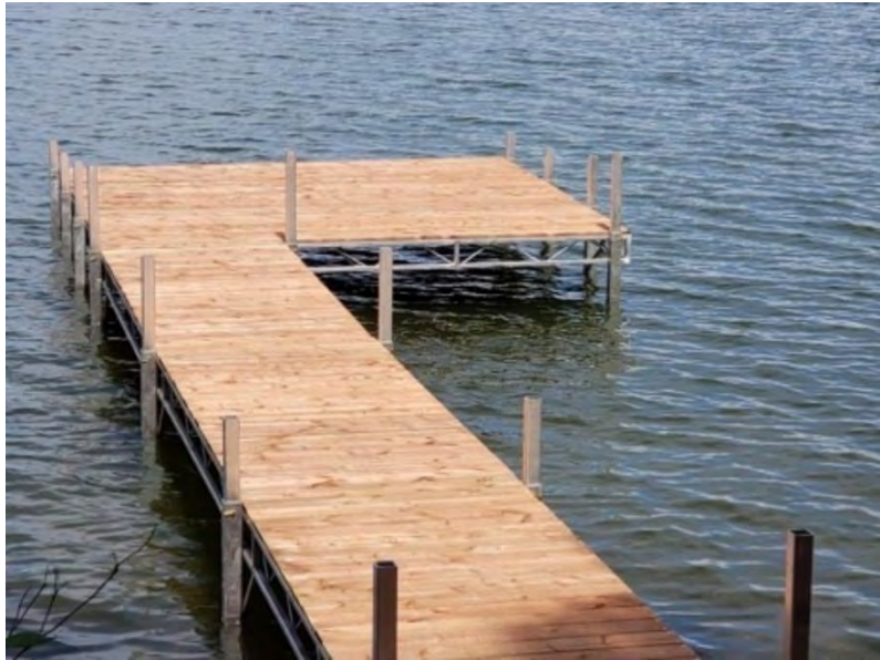
Figure 1 – Example of a wood deck rolling dock
