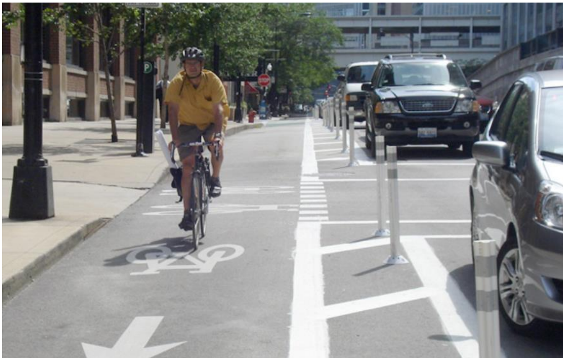
Figure 4.6: A One-way Protected Bike Lane using paint, bollard posts, and parked cars as protection from moving traffic.
