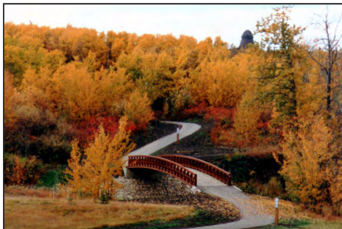
Pedestrian Bridge - Muskoseepi Urban Park
