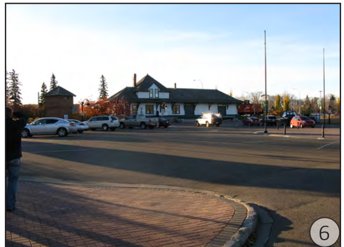
View of existing CN Railway Station looking towards 99 Avenue
