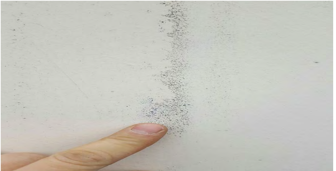
Top Coat Breakdown
